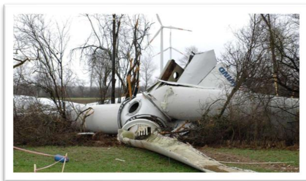
Figure 2: A wind turbine accident in Germany
