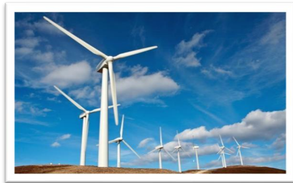
Figure 1: A 2 MW wind farm
